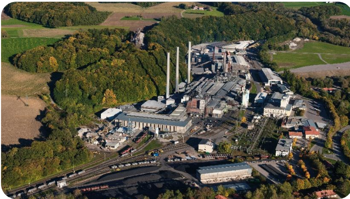
Aerial view of the Alzchem site in Hart with its three distinctive smokestacks. The smokestack on the right, which is about 100 meters high, will be carefully dismantled over the coming months.
